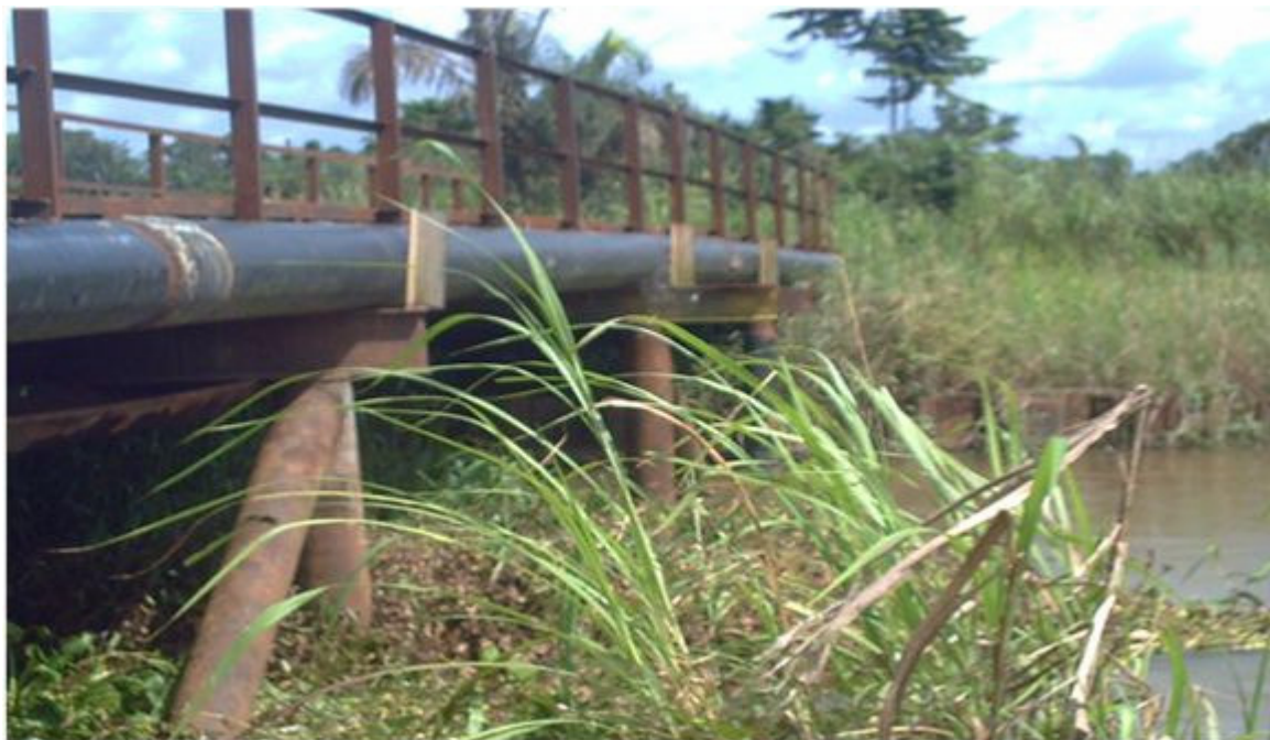
Plate 1. On-going metal construction work at sampling station 6.
