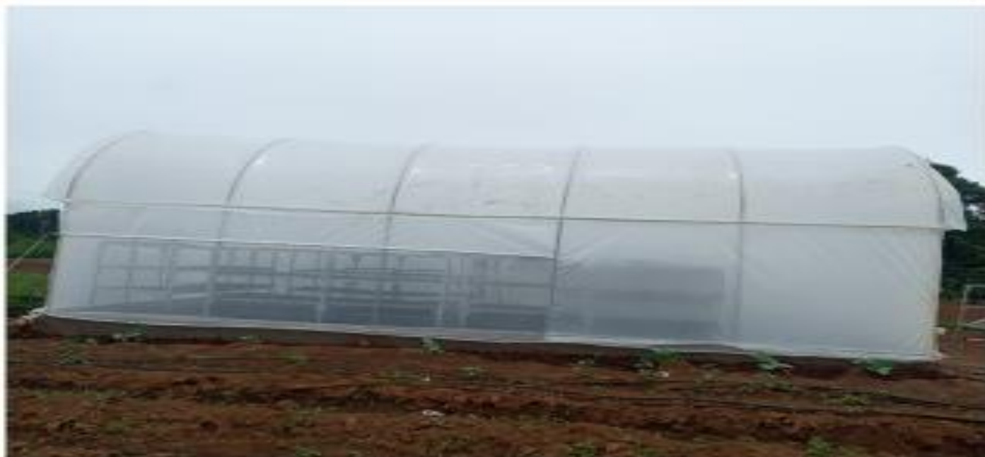
Figure 1 Solar Dryer House
