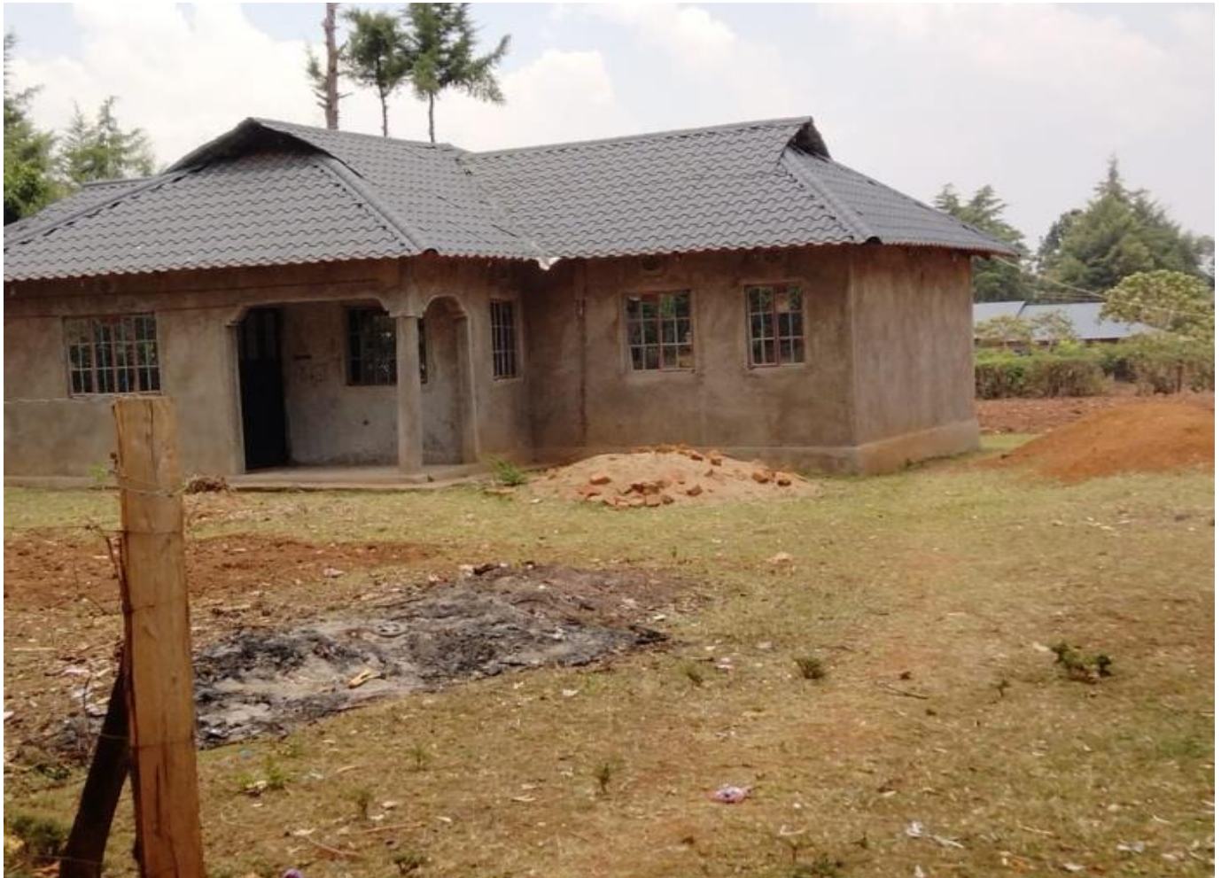
Residential House under Construction Indicating Peri Urban Land Use Change
