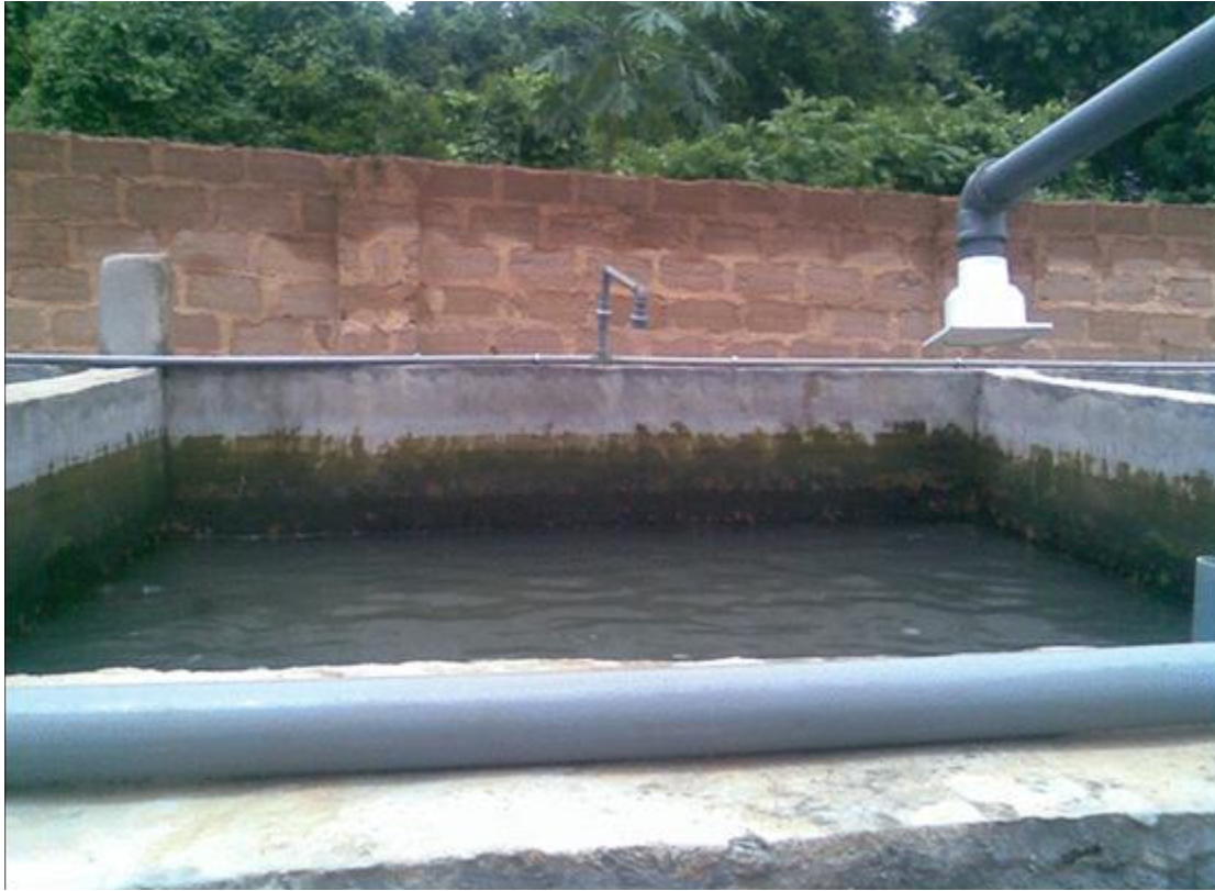
Plate 3. Concrete pond located in Iguosa.
