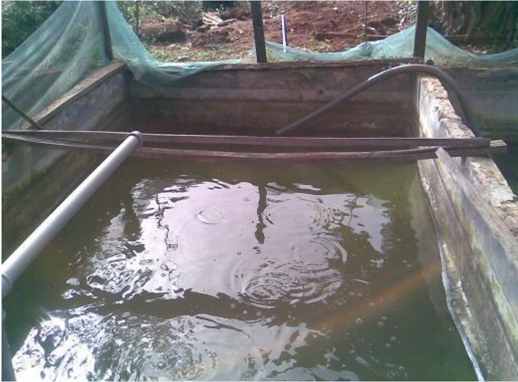
Plate 1. Concrete pond located in Oloku (1).
