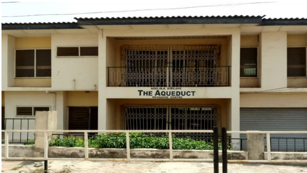
Fig. 3: The Aqueduct Resource Center at Old Bodija, Ibadan, Oyo State, Nigeria
