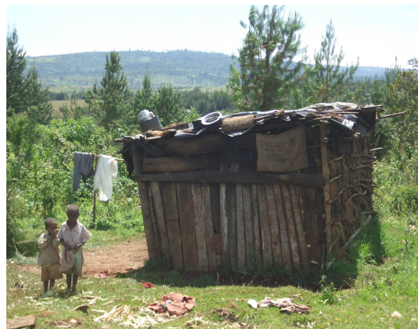
Figure 1: Mud/wooden walled house with polythene roof belonging to one of the study households
