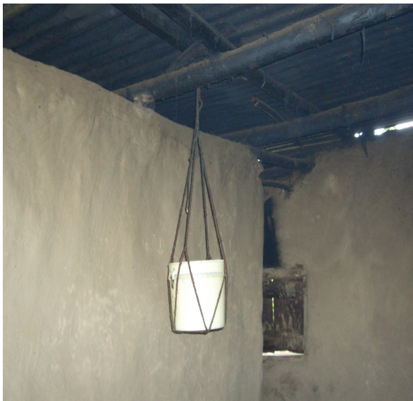
Figure 3: Ventilation in between wall and roof in one of the study homesteads
