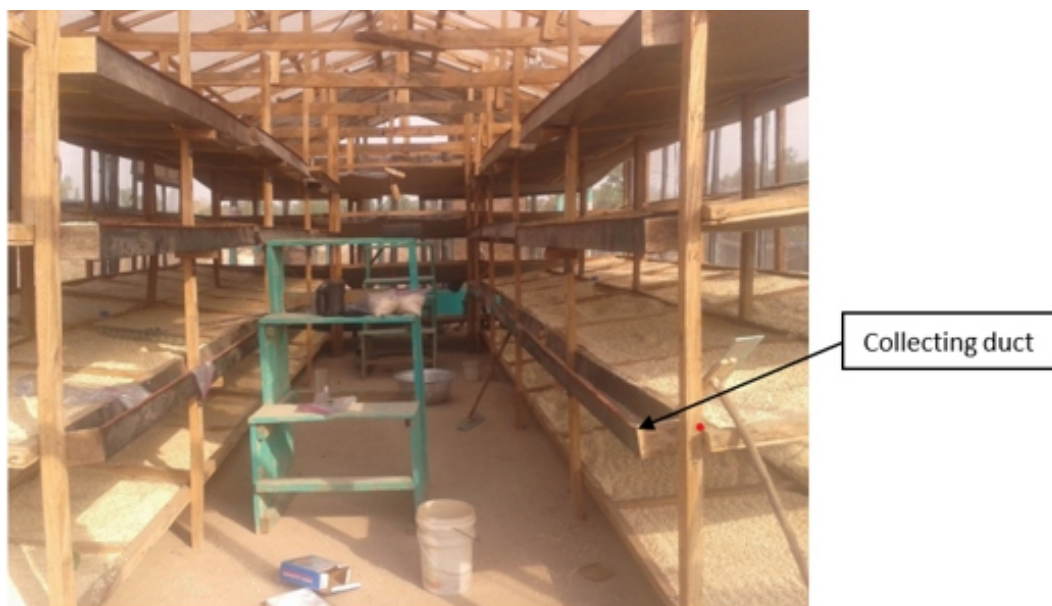
Figure 2: Inner view of drying chamber with shelves loaded with maize
