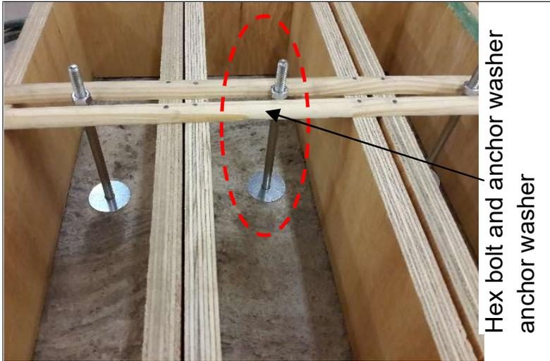
Figure 1: Timber box formwork
