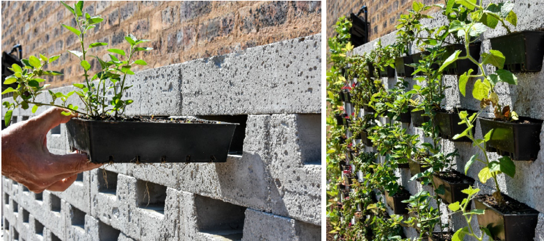
Figure 1: The Eco Green Wall has been custom-designed and manufactured in South Africa. It is a self-assembly system, which makes use of a commercially available low-cost soil tray and drip irrigation pipes that fit into the custom-made bricks. This allows for boundless size and shape assembly options.
