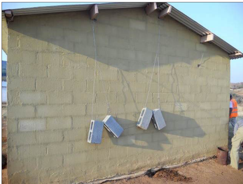
Figure 4: Typical roof anchoring system used for low-income houses
