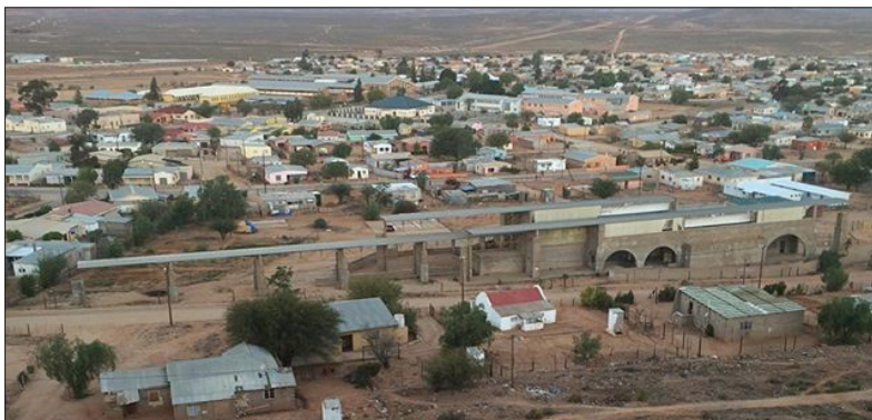
Figure 8: The context with the Steinkopf Community Centre in the foreground and another community centre in the background
