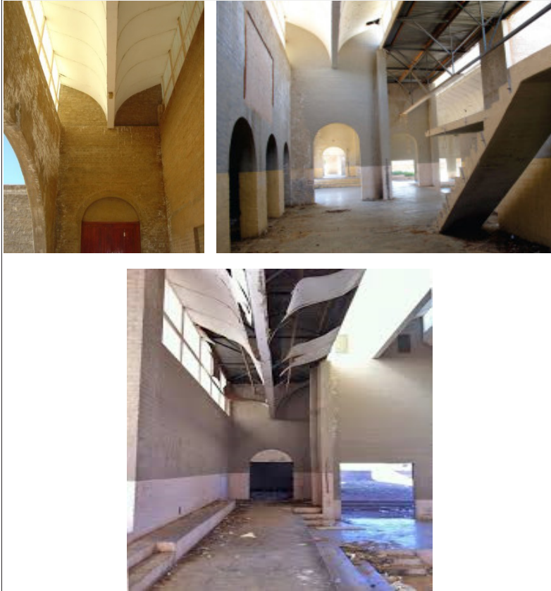
Figure 11: Steinkopf Community Centre, photo taken in 2007 (top) compared to recent photos of interior space in 2012 (bottom)
