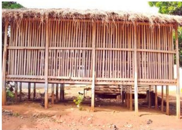
Plate 2. A raised platform used to store yam in northern Ghana.
