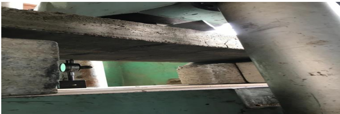
Figure 8: Failure mode of timber reinforced concrete slab
